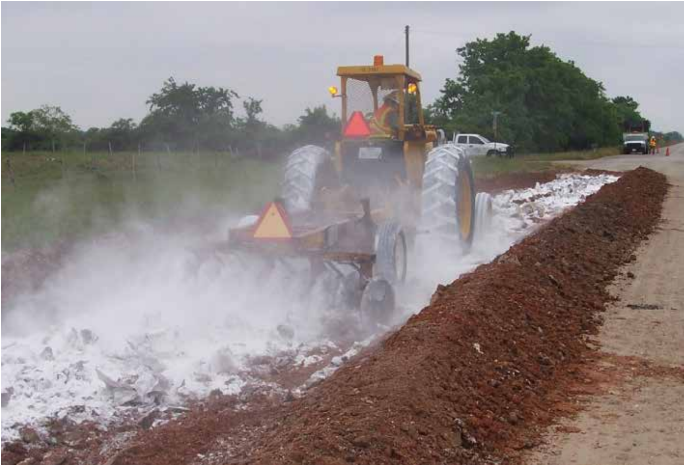
Figure 4-2. Lime Stabilization of Soil
