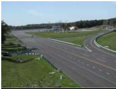
Award of Merit General Motors Proving Ground – ASTA Test Pad
