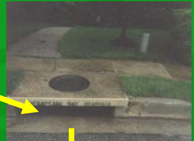
Storm Sewer Inlet
