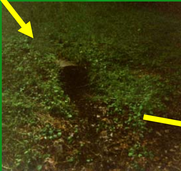
Storm Sewer Outlet
