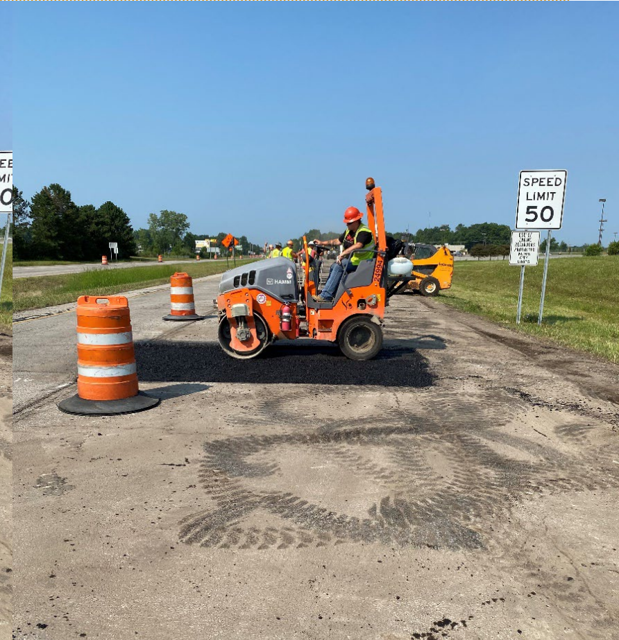
Small roller compacting asphalt in patch hole
