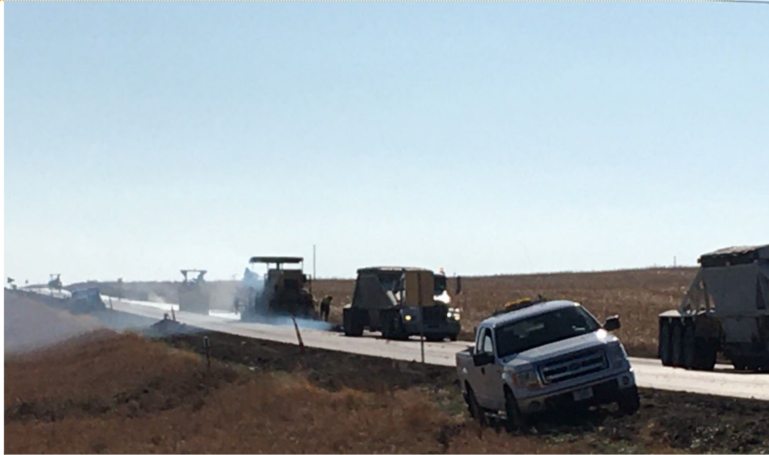
Paving train on State Highway 21
