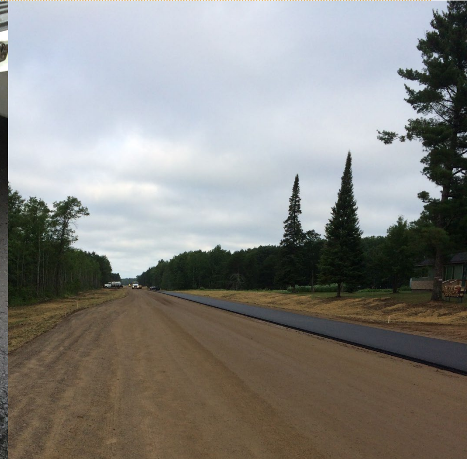
First lift on granular subgrade
