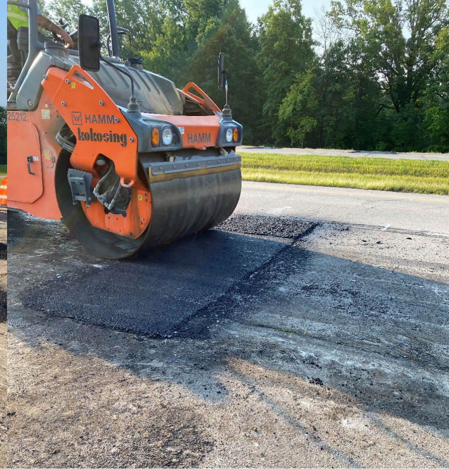
Roller compaction
