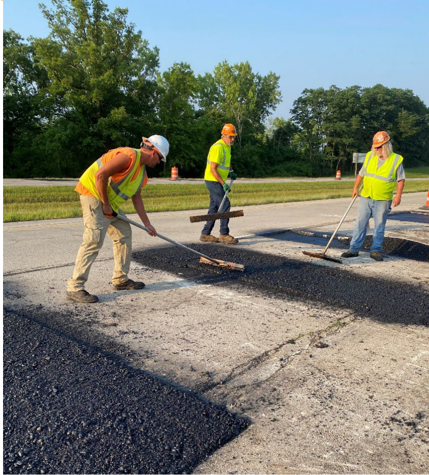
Final raking before compaction
