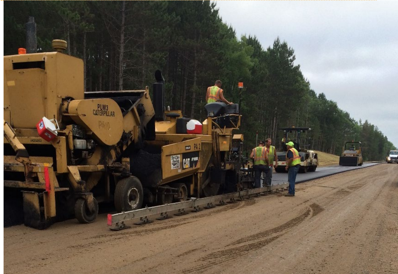
Paving on granular subgrade
