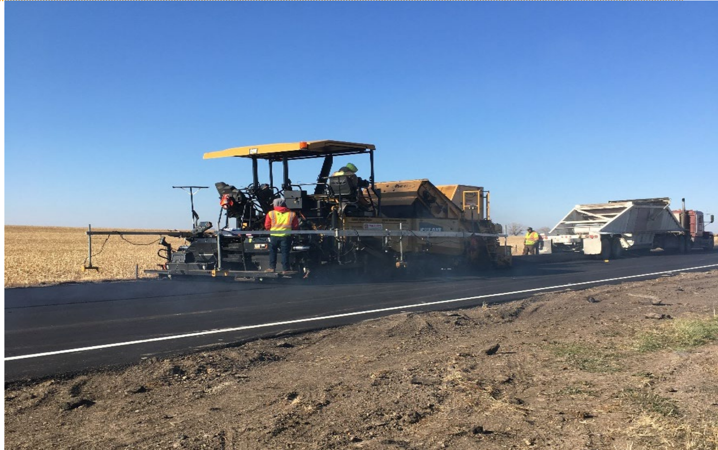
Paver, pick up device and truck
