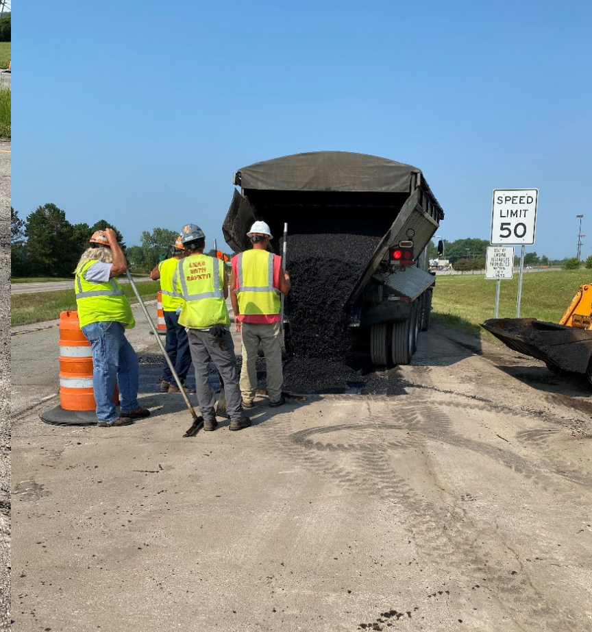
Dumping asphalt into patch hole
