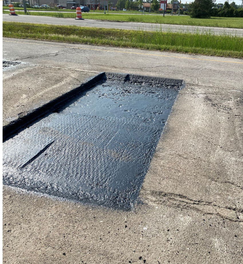
Tacked patch hole ready for hot mix asphalt
