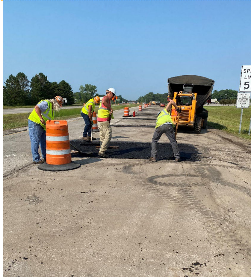
Construction crew shoveling and raking asphalt throughout patch
