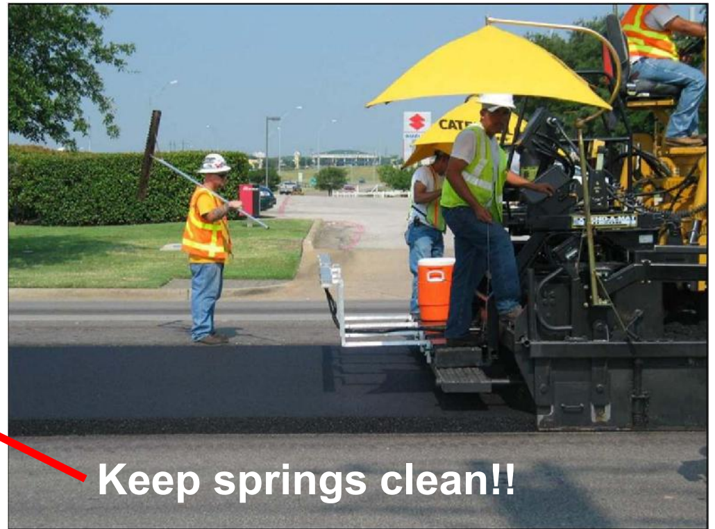
CORRECT SQUARE JOINT — END GATE DOWN
