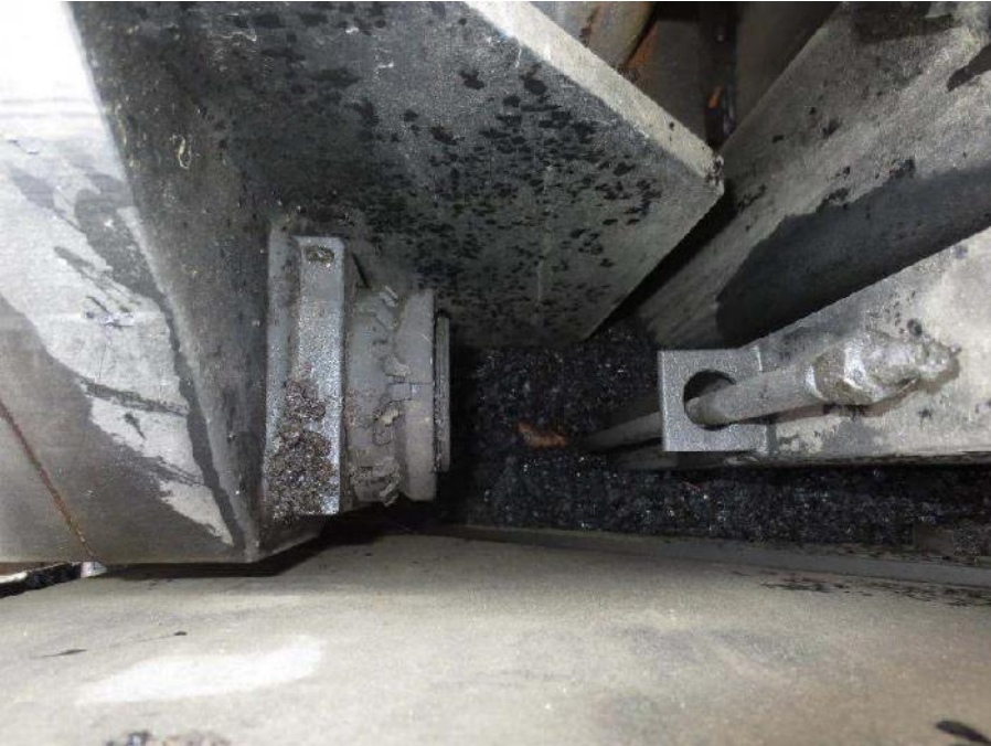
View looking down on top of pivot point
