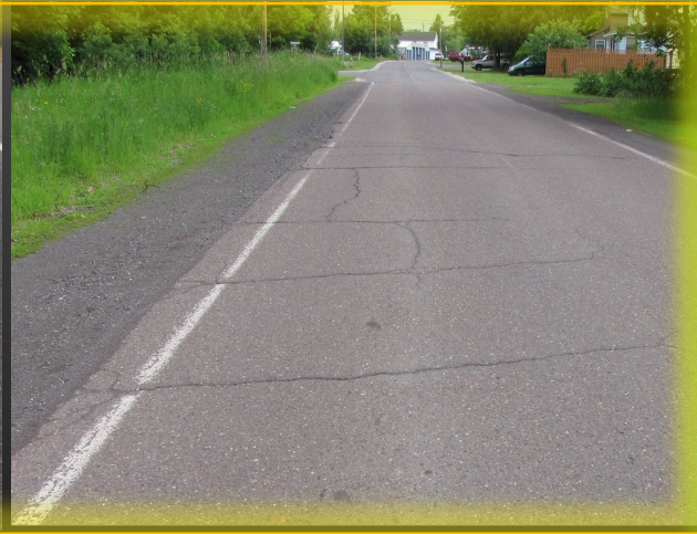
Block Crack
