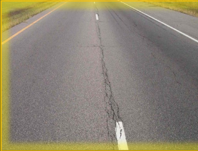
Joint Crack
