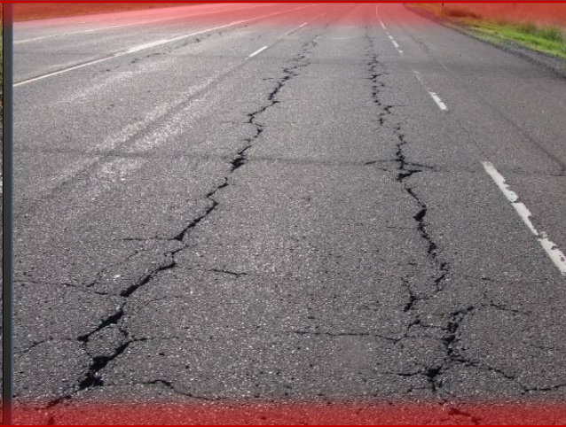
Shear Crack
