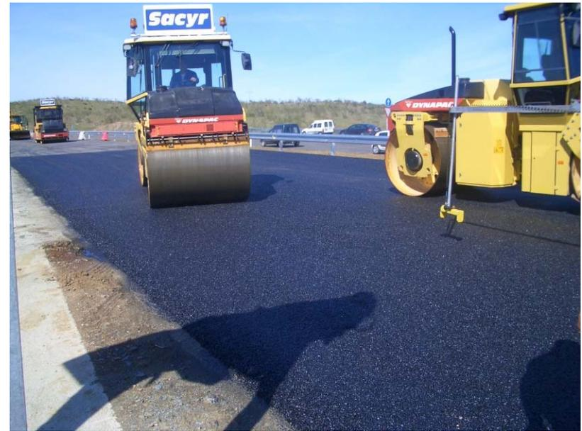
Differing temperatures at compaction means differing density – differing service life
