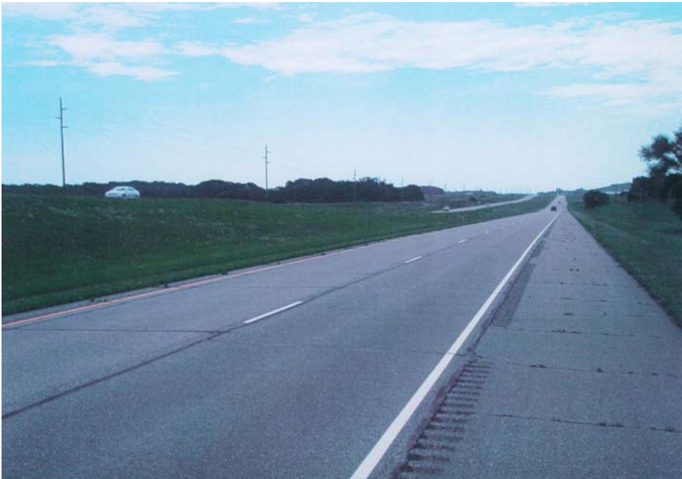
The Minnesota Department of Transportation won a 2009 Perpetual Pavement Award for the eastbound lanes of US TH 10, east of Detroit Lakes to east of Perham.
