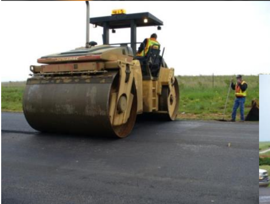
Rolling Transverse Joint
