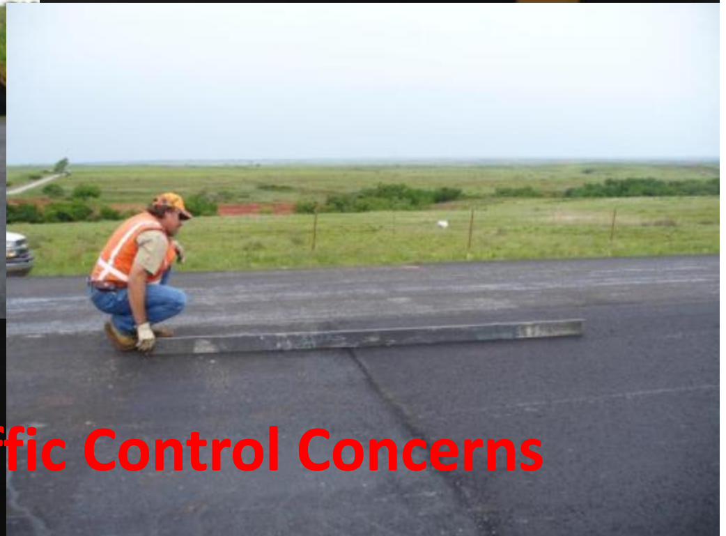
Checking Transverse Joint
