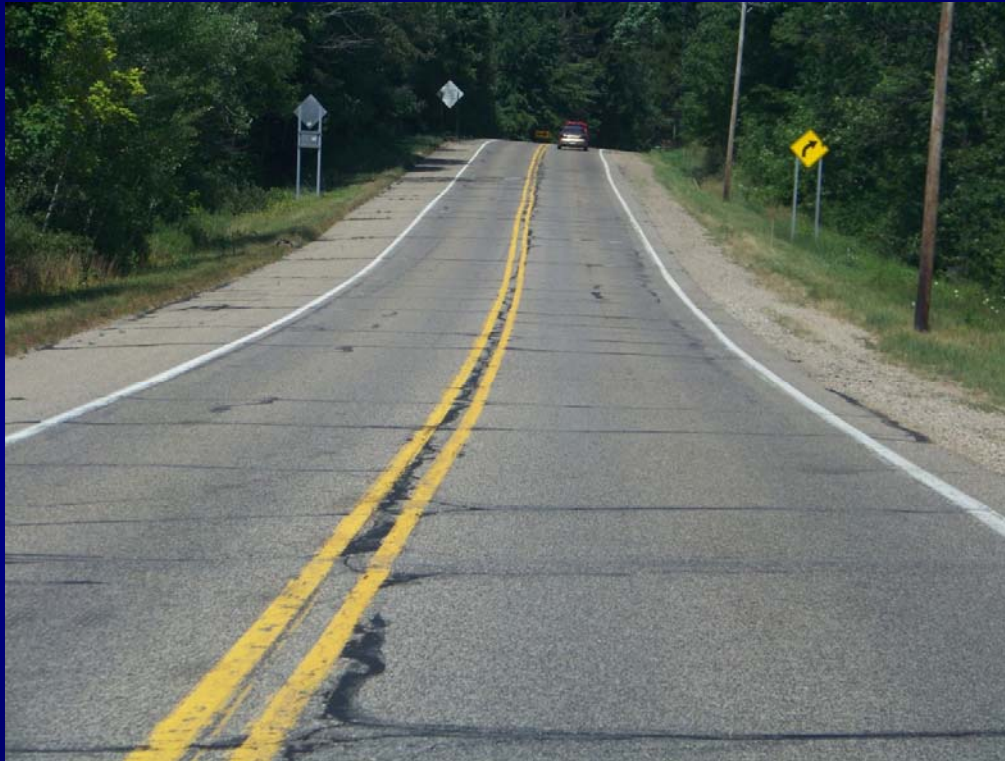
M-21, Before Construction
