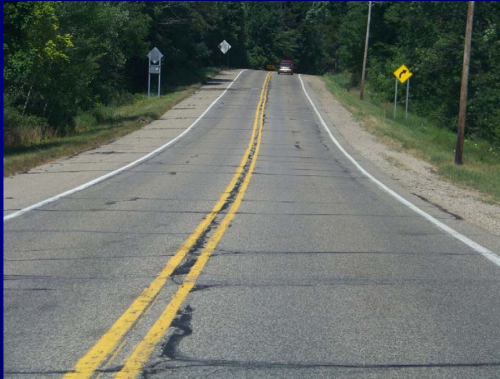
M-21, Before Construction
