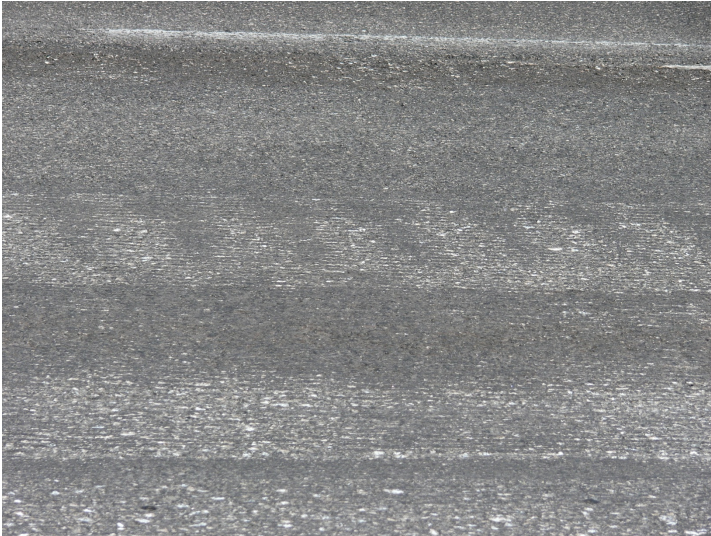
Scalloping due to excessive foot speed
