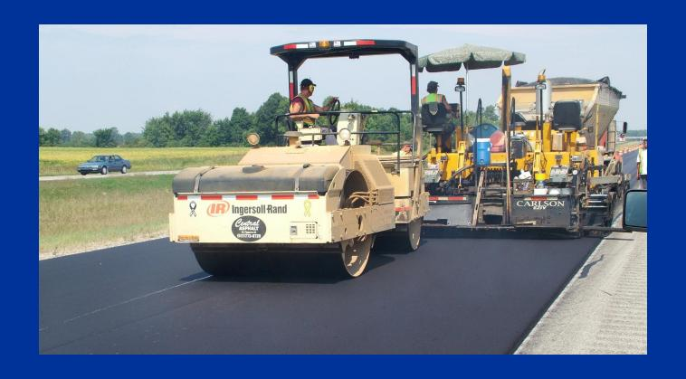
One of the Essentials for a Consistent and High Quality Asphalt Pavement is to Provide for a Continuous Operation
