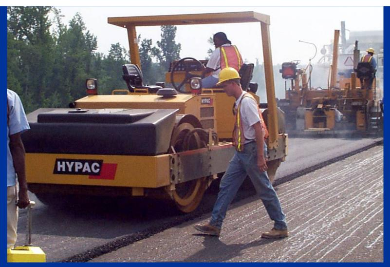
If everything else is unchanged, roadway performance will be a function of construction compaction
