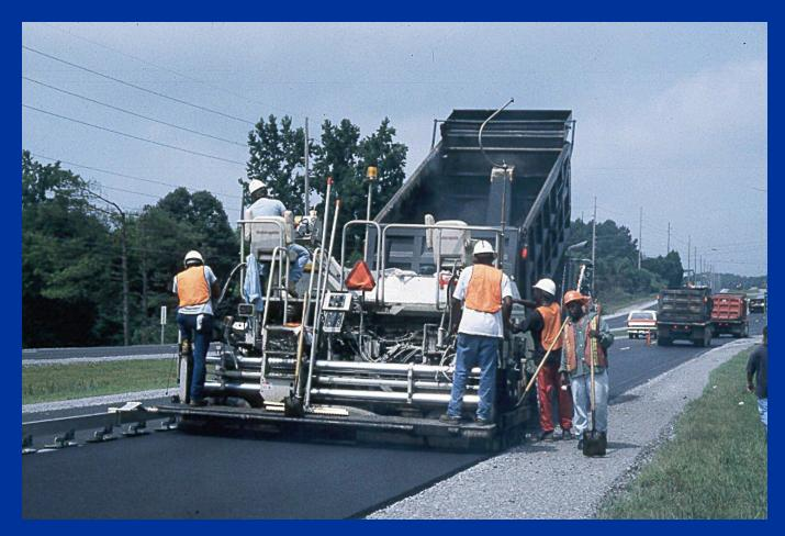
Rule of Thumb: the HMA density behind the screed should be about 85% of Gmm (85% Density)
