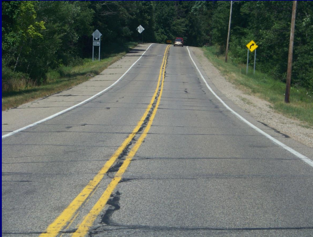
M-21, Before Construction
